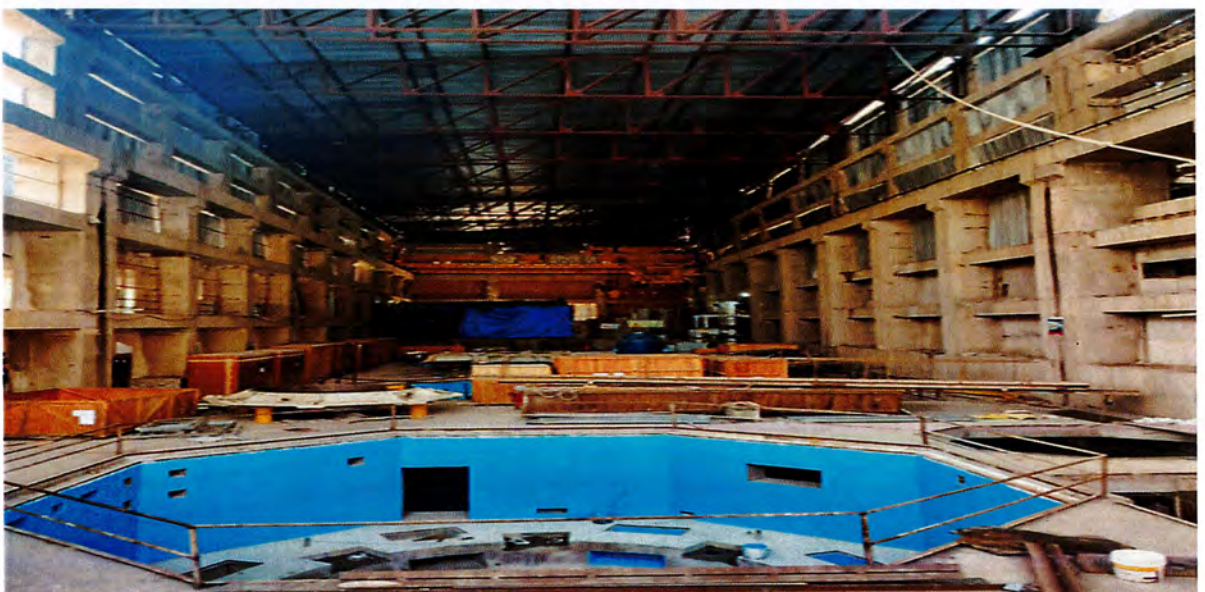
SURFACE POWER HOUSE UNDER CONSTRUCTION - 120 MW RANGIT-IV (SIKKIM)
