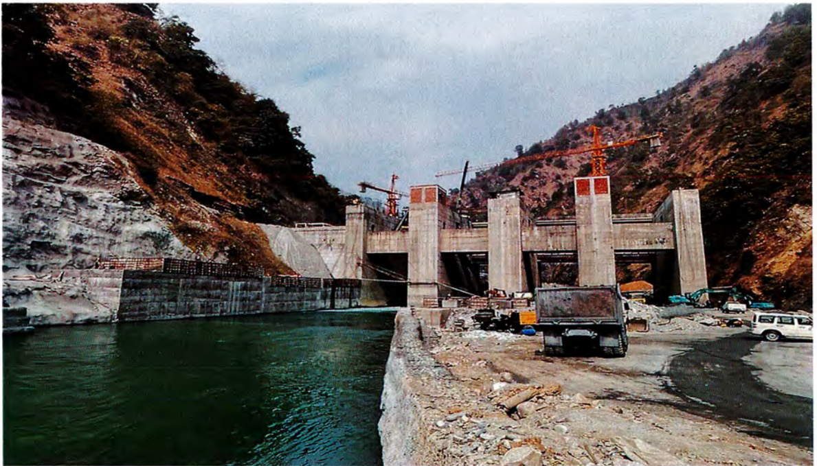
D/S VIEW OF DAM (AFTER RIVER DIVERSION)
